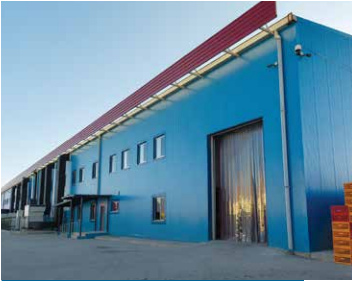
Water Gutters, Down Take Pipes
