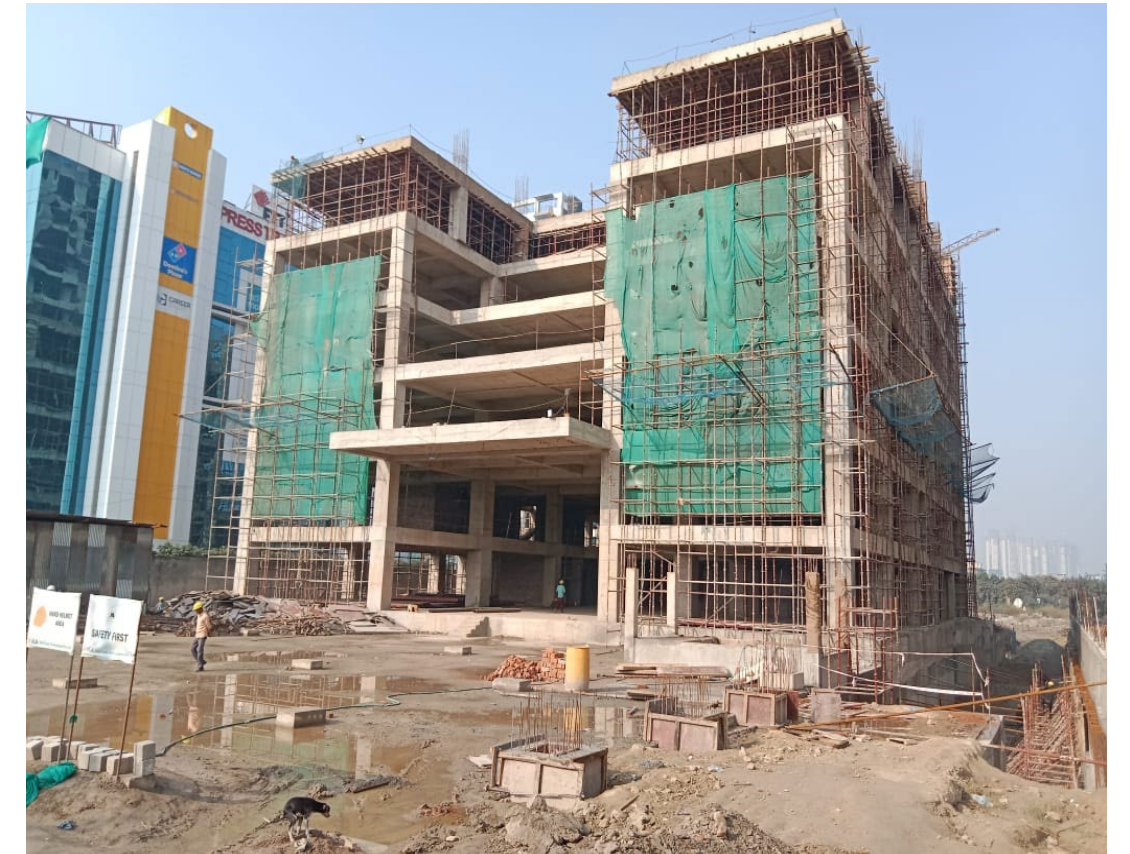
APL Apollo new Corporate office (Work in progress)
