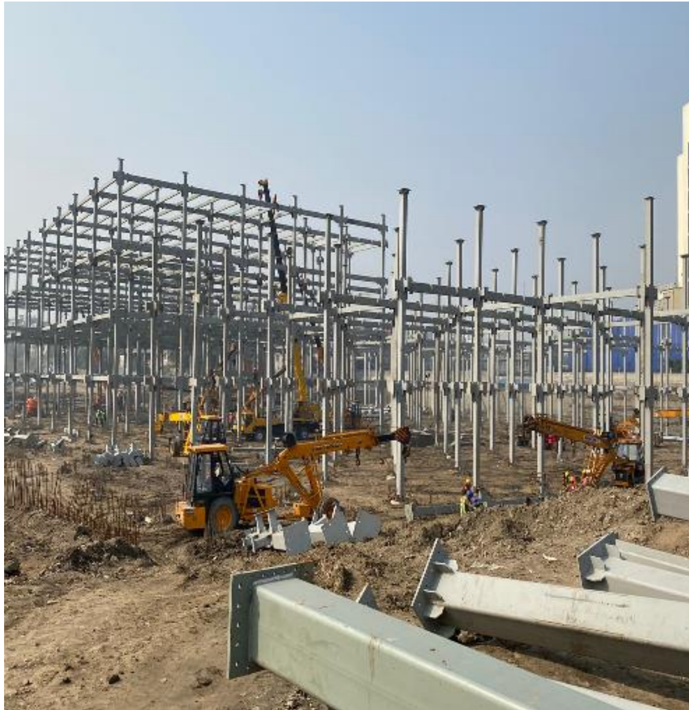
Hospital structure put in place in 6 weeks
