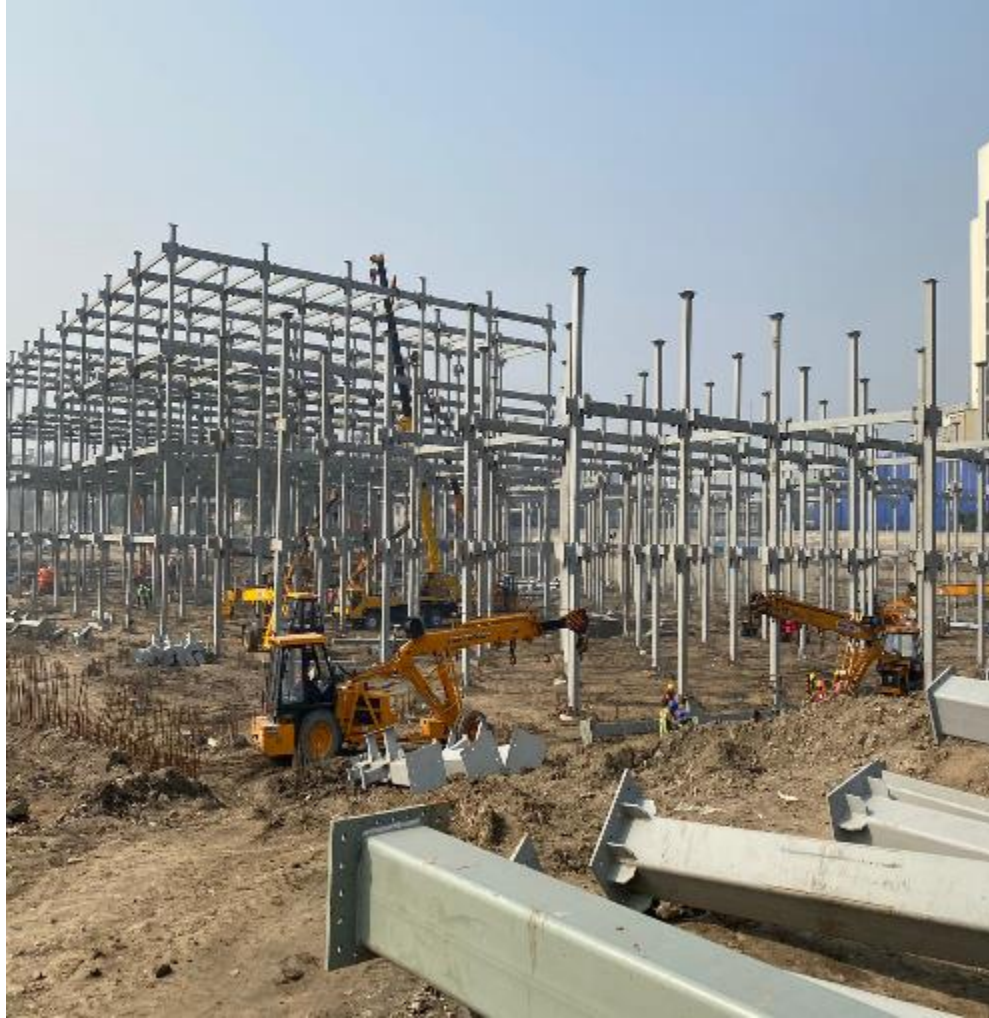
Hospital structure put in place in 6 weeks
