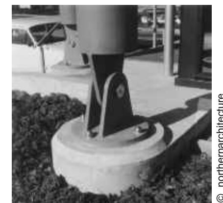
Some examples of HSS connections with pinned ends
