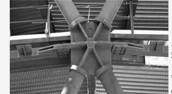
Moment - resisting connection is achieved by a welded end- plate with four or more bolts. The thickness of the end plate depends on the moment to be transferred
