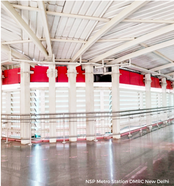
NSP Metro Station DMRC New Delhi
